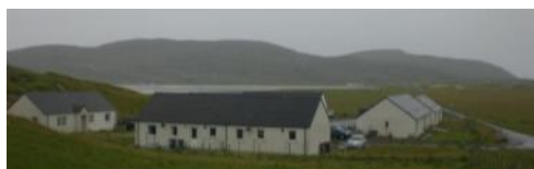
3 Units at Cialla, Eoligarry, Barra
