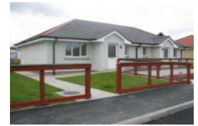
12 Units at Arras Cottages, Perceval Road, Stornoway,
