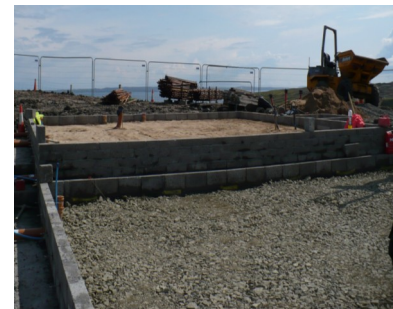
4 houses at Cnoc A'Runaire, North Tolsta
