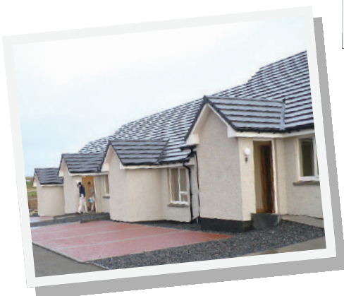
4 houses at Cnoc A'Runaire, North Tolsta
