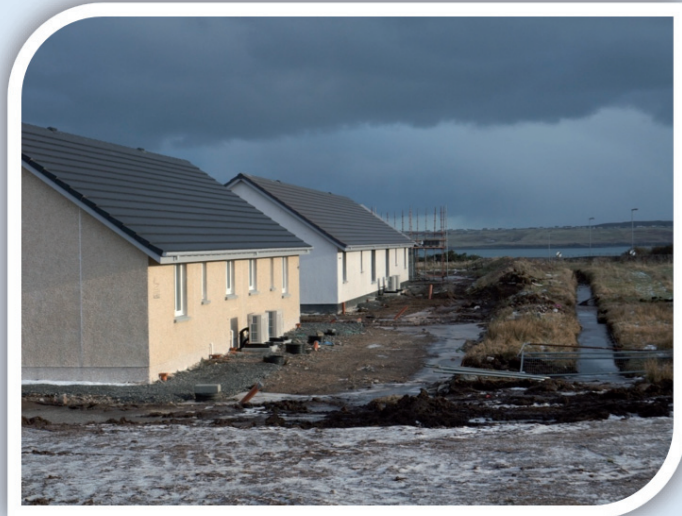
Mackenzie Crescent, Sandwick, Isle of Lewis
