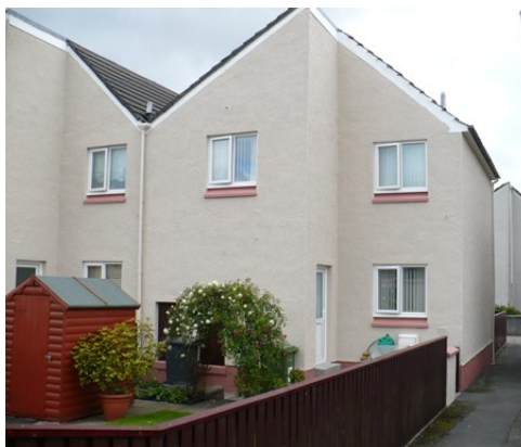
Painterwork at MacLennan Place
