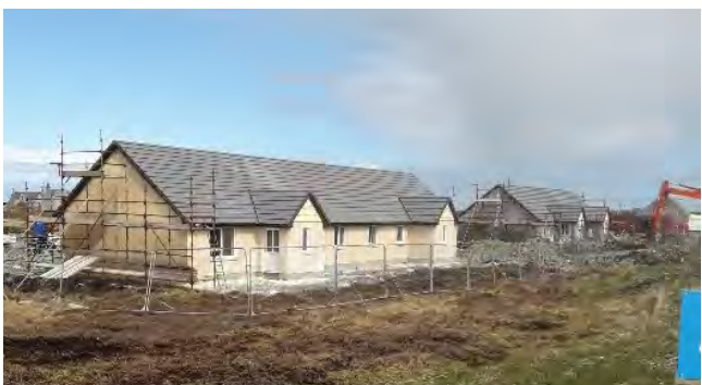
Alex Murray Construction are on site at South Dell, Isle of Lewis, constructing 6 new homes for social rent
