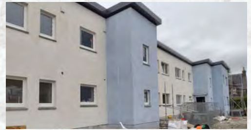
Alex Murray Construction continues work on site at the former Police Station, Tarbert. The flats are scheduled for completion in October 2021.
