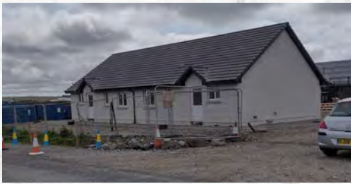
Calmax Construction are progressing well at the 8 homes site at Barvas now named Gleann Mor.
