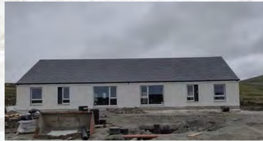
Macinnes Brothers are progressing on site at Howmore named Ionad Mairi Bremner to build 4 homes for social rent.
