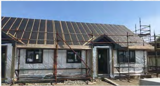
Work is ongoing at the Low Flyer site at Balivanich by Calmax to provide 10 homes for social rent.
