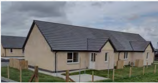
Alex Murray Construction have completed the site at South Dell, named Sealladh Beinn Dail, constructing 6 new homes for rent.
