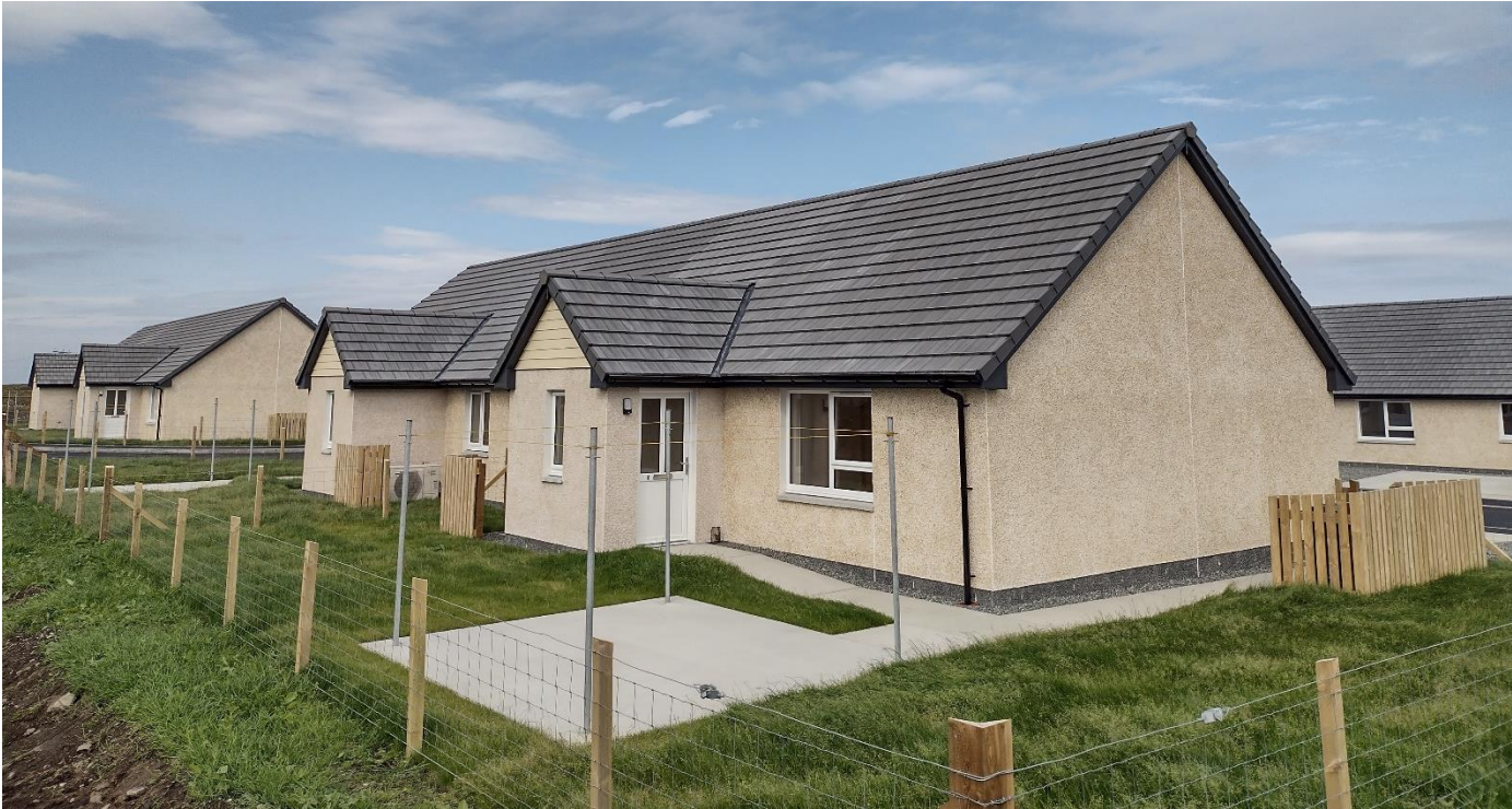
South Dell – Alex Murray Construction
