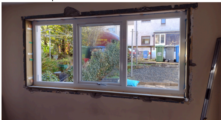
New windows being installed in the Cearns
